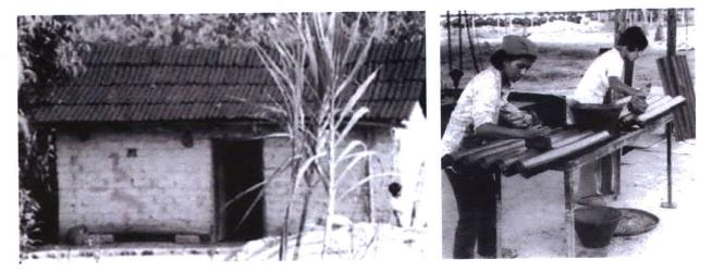
Figure 4.8: Corrugated Asphalt Roofing Sheets (ARS) made with natural fibres and hot paving grade asphalt. Images from BASIN pamphlet on roofing, Shelter Forum, Nairobi, Kenya.
