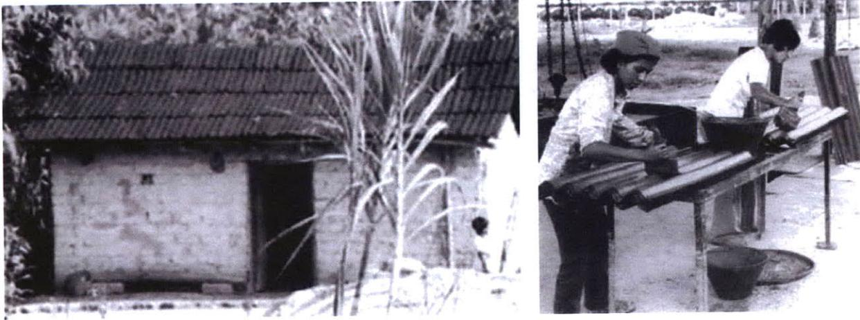
**Figure 4.8:** Corrugated Asphalt Roofing Sheets (ARS) made with natural fibres and hot paving grade asphalt. Images from BASIN pamphlet on roofing, Shelter Forum, Nairobi, Kenya.
