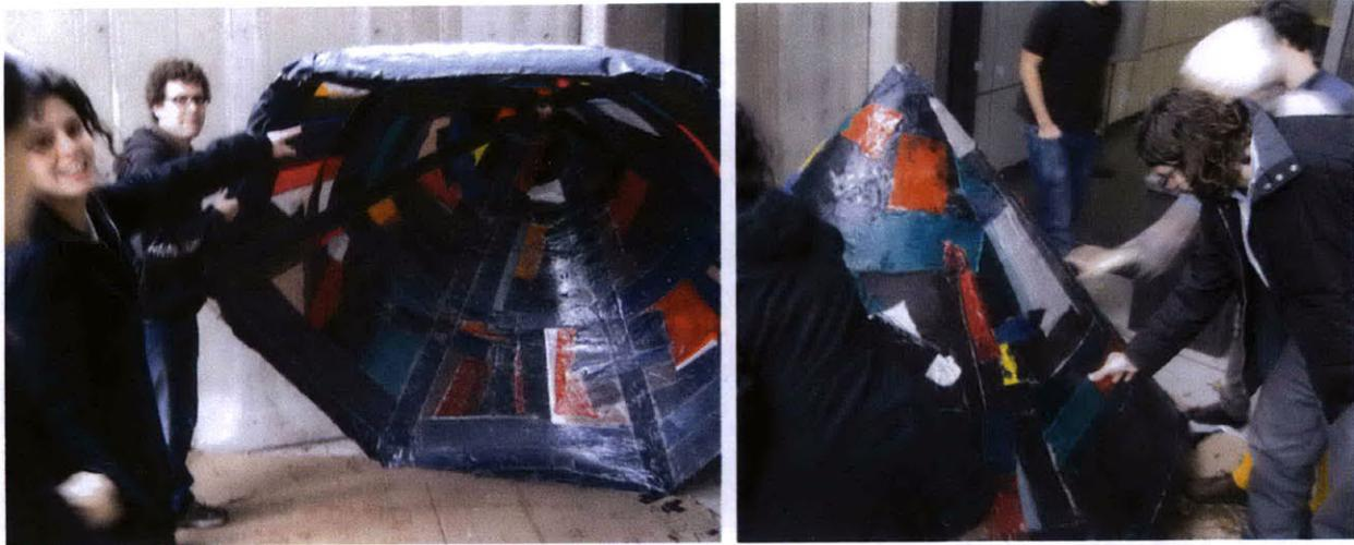
**Figure 7.9:** David Robert, David Cranor and Edwina Portocarrero built an inflatable mould which they used to lay up recycled apparel fabric with epoxy resin.
