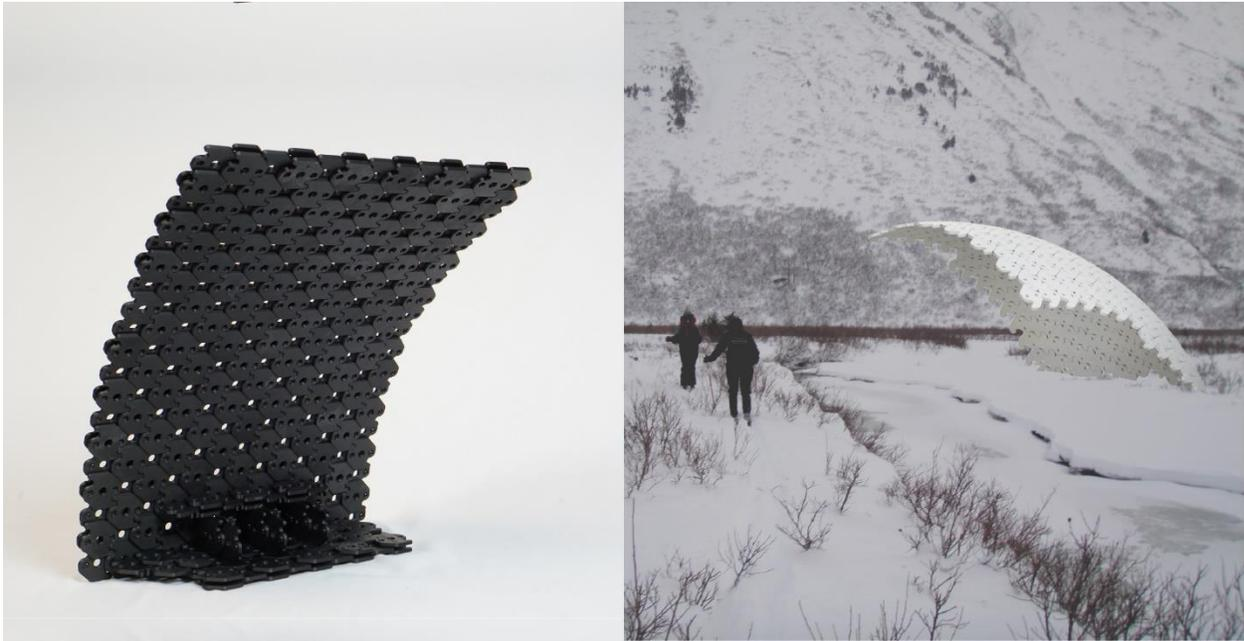
Figure 74 Concept for a potential structure utilizing the play between the parts to form a curved canopy.
