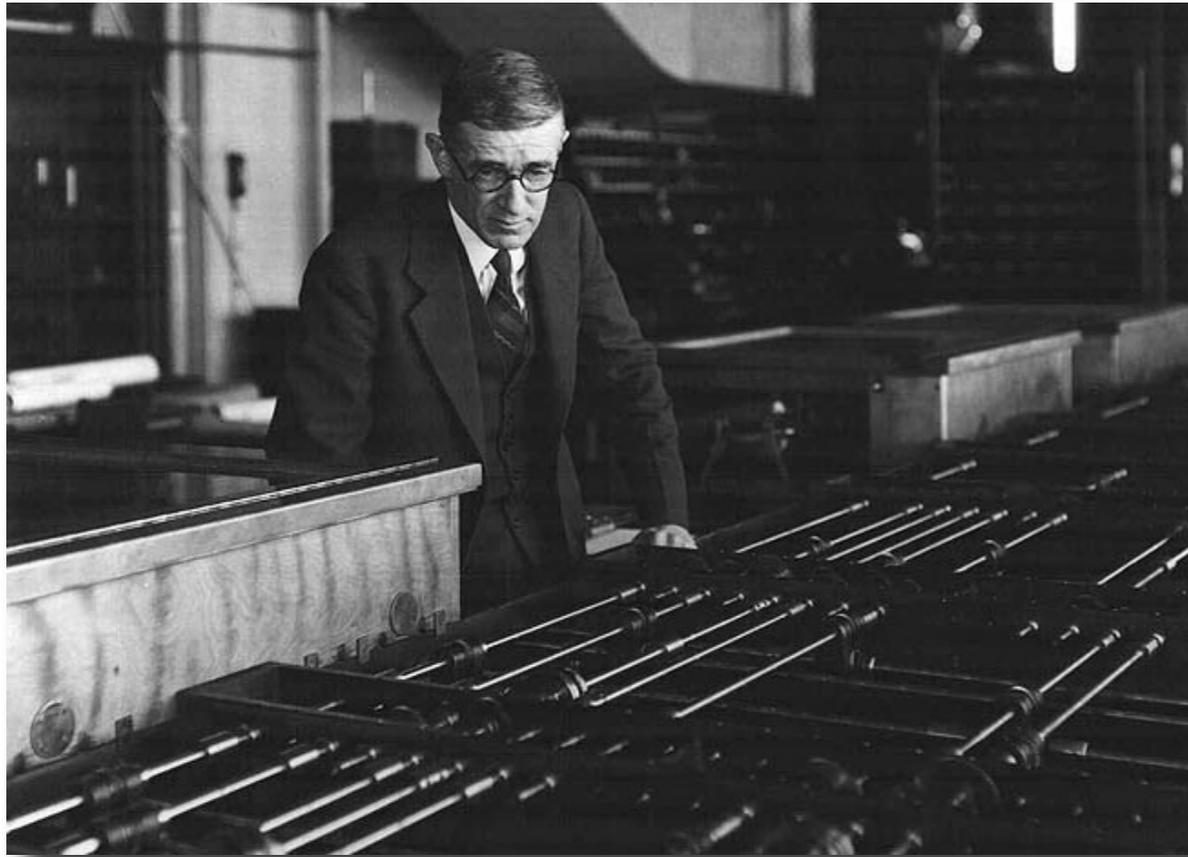
Vannevar Bush and Differential Analyzer, MIT, 1931
