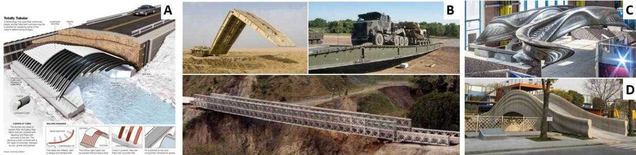
Figure 4-1: State of the art advanced bridge technologies. A) CFRP tubes which arguably can fit “in a backpack” [111], B) rigid deployable bridges [112], C) Wire-feed metal 3D printed bridge [14], D) layer-based deposition concrete bridge [113].
