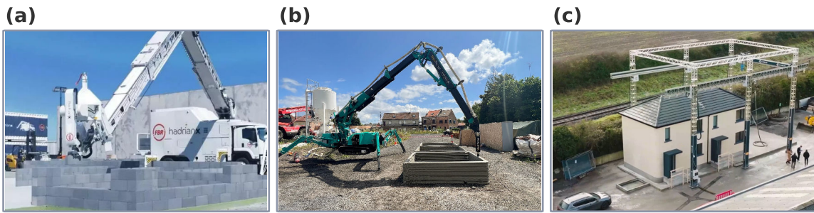
Figure 1.1: Robotic construction systems in which the machine is larger than what it builds. (a) Hadrian X, a truck-mounted bricklaying robot [5]. (b) MaxiPrinter, a mobile 3D concrete printing robot [7]. (c) gantry-based 3D concrete printing of housing [8]. Images: manufacturer and press material, as cited per panel.
