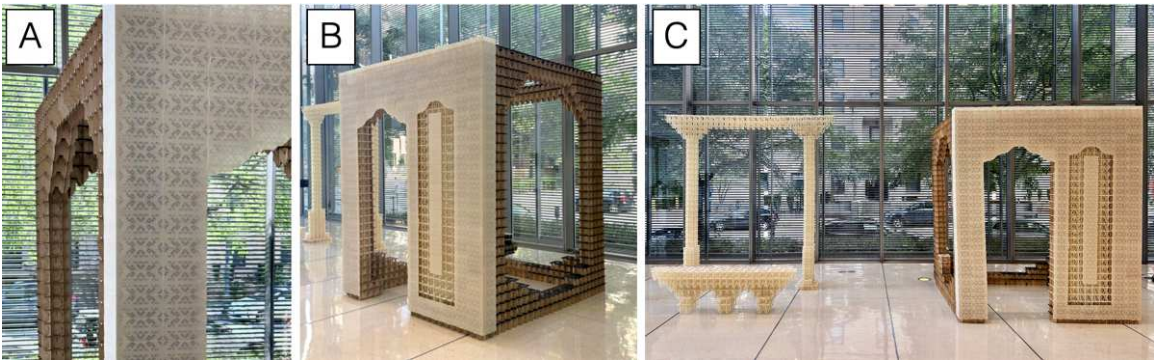
Figure 6-30: A) Detail view of bioplastic cladding with decorative Bhutanese inspired geometric design. B) Front of the the tiny house with example cellular cladding. C) Archway and bench next to house. Photos from Vlasta Kubusova.
